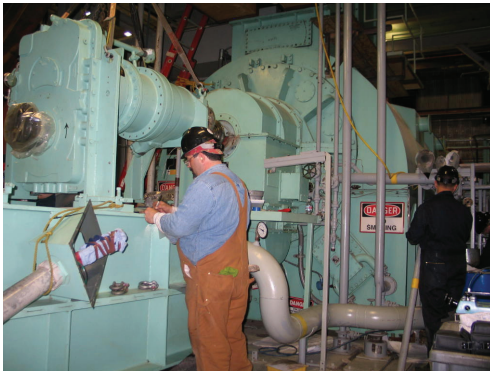
Chugach and ML&P are proposing to partner on a new Anchorage power plant.
