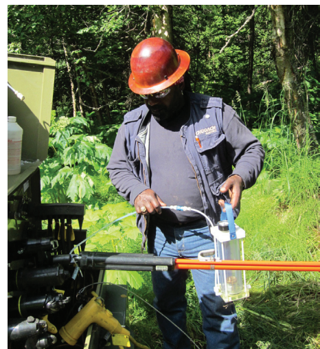
Injections can extend the life of underground cable.
