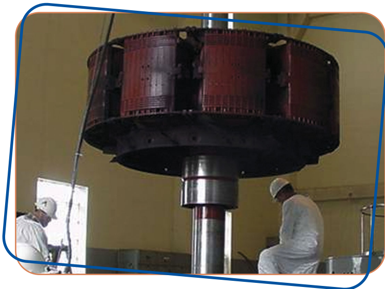
Cooper Lake Hydroelectric Plant
