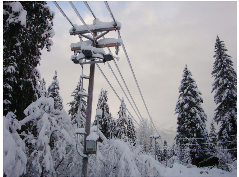
Heavy snow loading on conductors and trees contributed to outages in Girdwood and Indian in late December.
