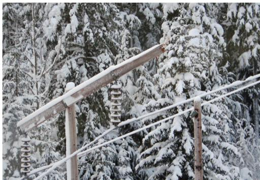
Heavy ice broke a structure and brought wires to the ground on the 115-kv line a few miles north of Cooper Landing in late December. The remote location made repairs difficult. Crews needed snowmachines to get to the site, and a helicopter to fly in replacement parts.
