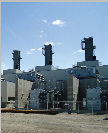
The first-firing of gas turbines at the Southcentral Power Project took place in mid-October as part of the commissioning process for the new power plant. SPP is expected to begin commercial operations the first quarter of 2013.
