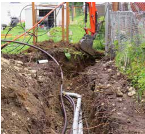
An overhead-to-underground conversion project is underway near Cheney Lake.
