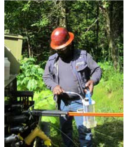
Cable injections can add years to the life of underground cable without digging up neighborhoods.
