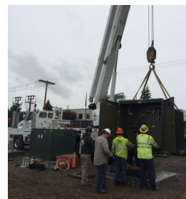
Unloading power transformer
