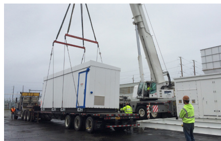
Power Control Module
