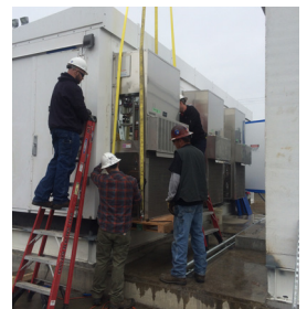
Installing air condition unit on flywheel module
