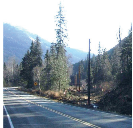
Chugach is relocating 3.5 miles of distribution line nearer the Hope Highway to make it easier to find and repair problems.
