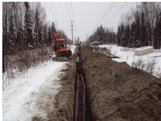
A project is underway along tudor road to convert 1.5 miles of overhead distribution line to underground.
