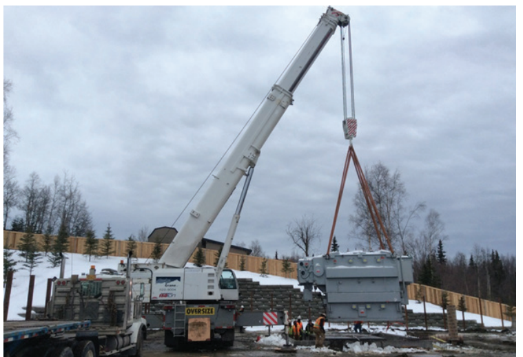
The transformer for the Hane Substation was placed on its foundation in late November.
