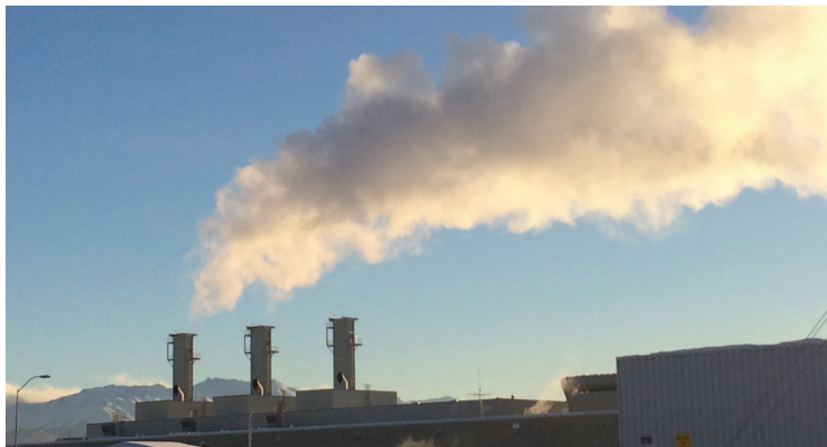
While the efficient, new Southcentral Power Project has been running around-the-clock throughout the year, colder winter temperatures make the small amount of water in its emissions visible.
