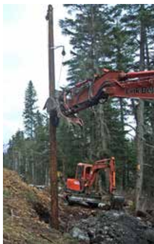
Crews set a new pole as a part of the relocation of a mile of the Hope line.
