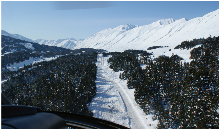
Chugach rebuilt 15 miles of transmission line through Turnagain Pass this winter.
