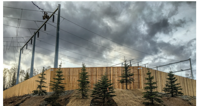
Fencing and landscaping at the new Hane Substation.
