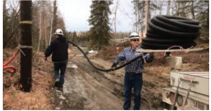
The Corflo Reel allows crews to work safely and more efficiently.
