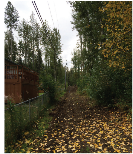
This photo shows a section of easement where the new underground line was installed prior to converting services for the homes on the left, and retiring the existing overhead power line. Park land, heavily forested with cottonwood trees, borders the right side of the easement.
