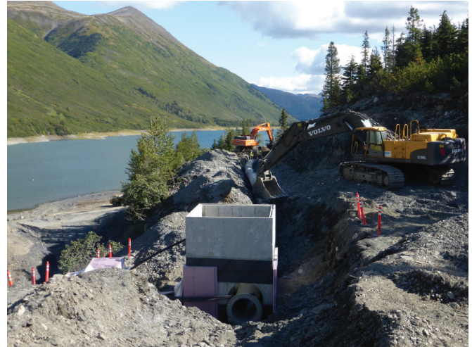
Substantial completion of the Stetson Creek diversion project at Cooper Lake is expected by mid-December.
