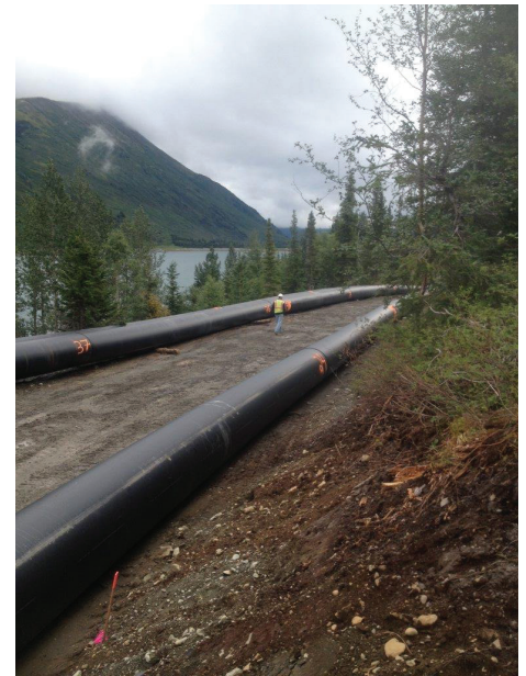
Two miles of buried pipe will carry water from Stetson Creek to the Cooper Lake reservoir.
