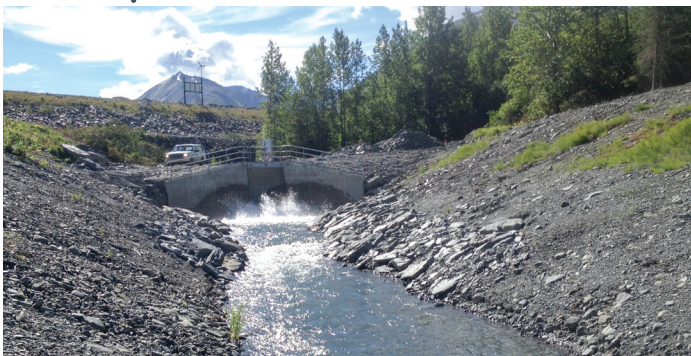
The Stetson Creek diversion project allows water from the Cooper Lake reservoir to be released to Cooper Creek.
