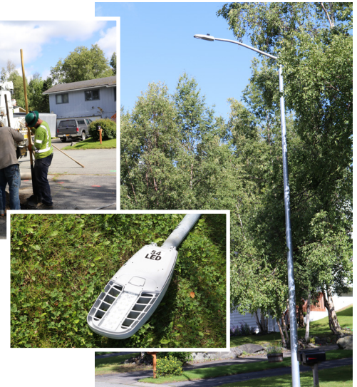
New streetlight pole and a more efficient 54 watt LED fixture being replaced by Chugach crews.
