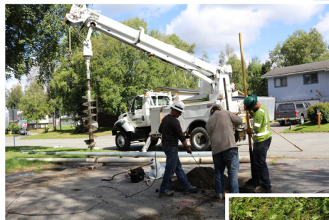
New streetlight pole and a more efficient 54 watt LED fixture being replaced by Chugach crews.
