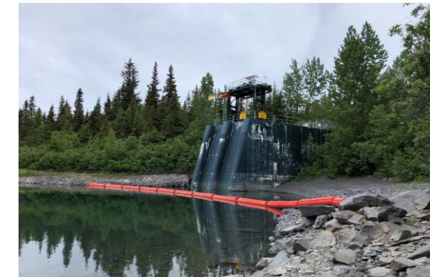
COMPLIANCE – COOPER LAKE REGULATORY & DAM SAFETY $181,000
