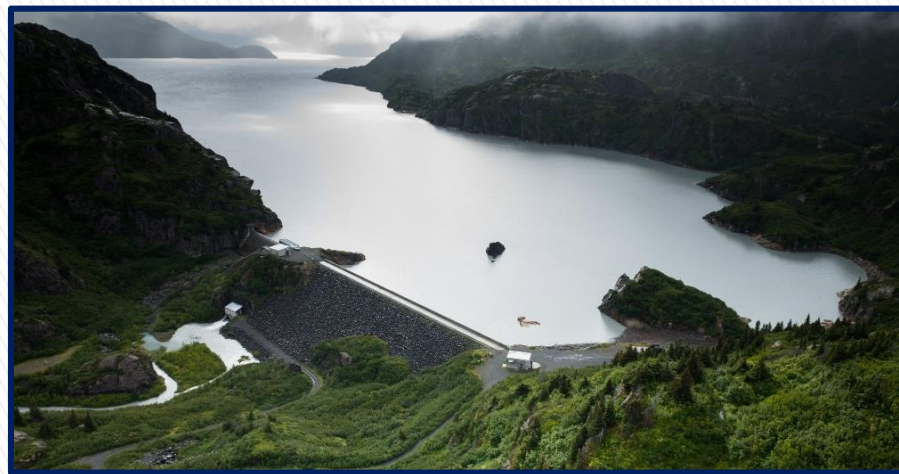
Bradley Lake Hydro Project
