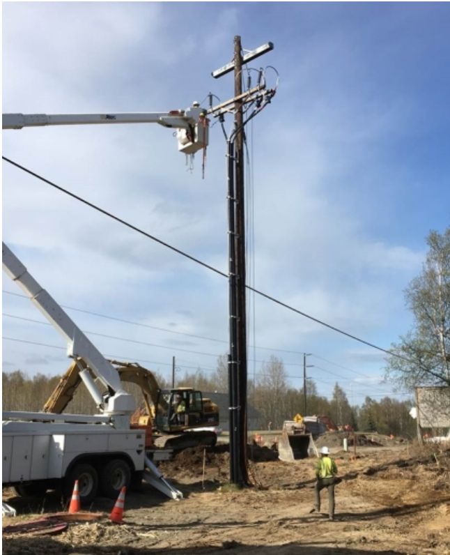
Installing 34.5 kV Riser
