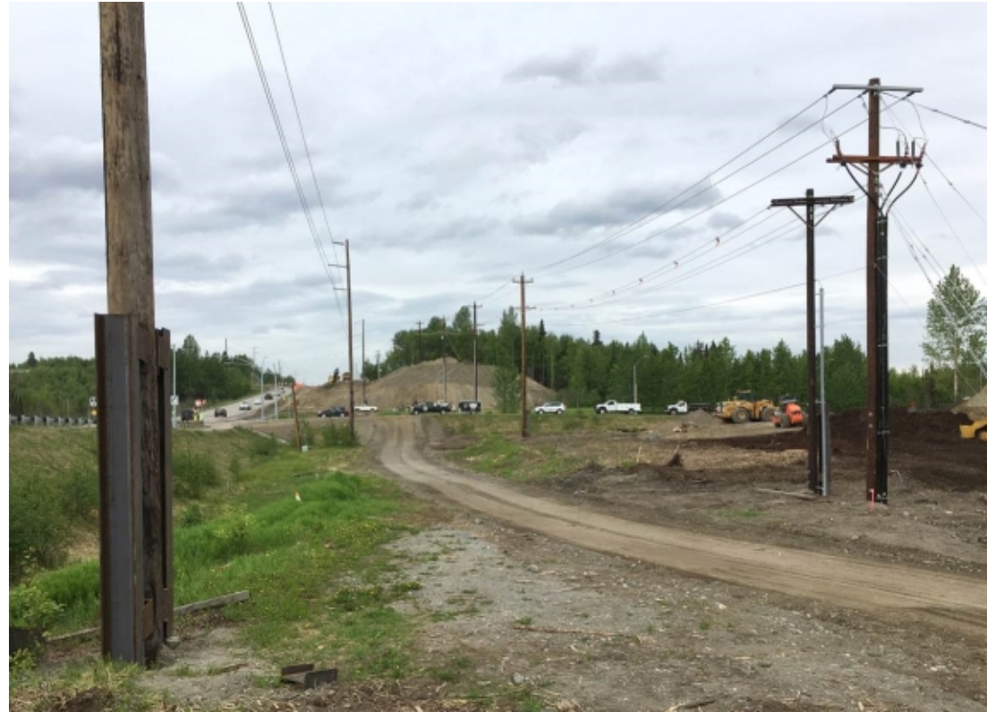
Temporary Relocated 34.5 & 12.5 kV Lines
