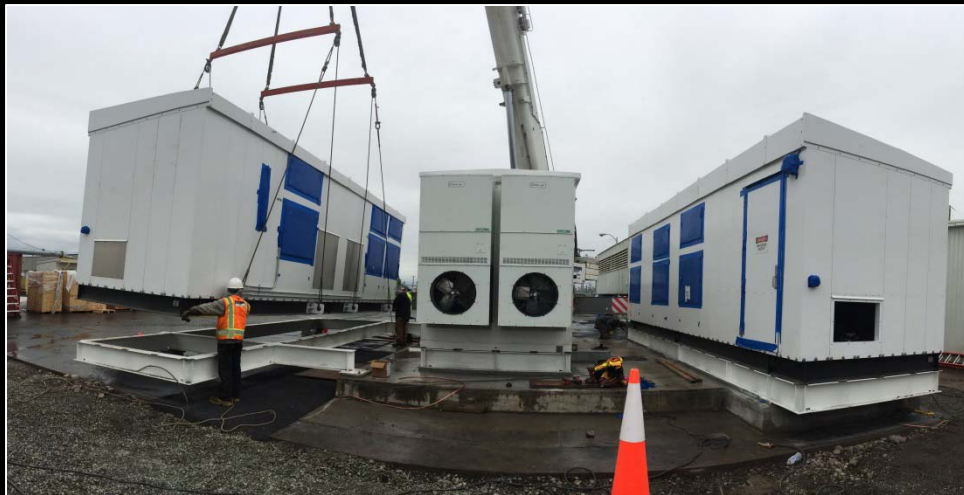
Battery PCS enclosure being set on foundation
