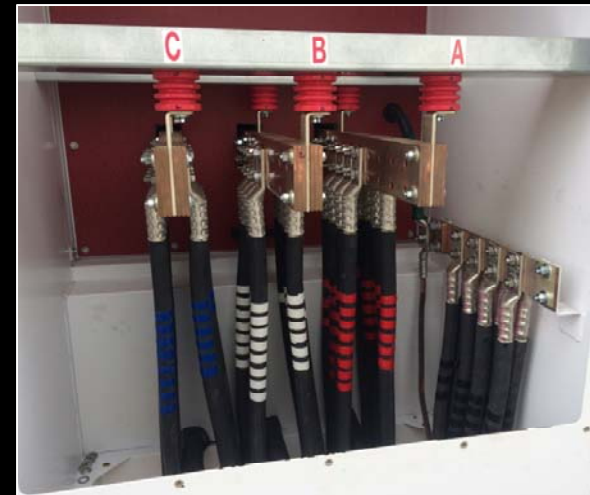
BESS AC Termination Cabinet
