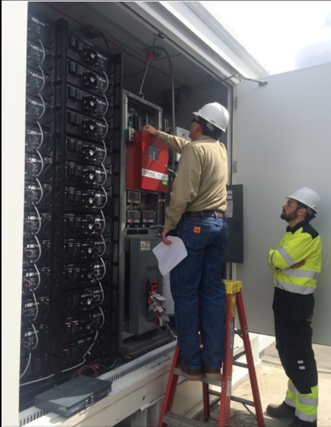
System check in the BESS enclosure
