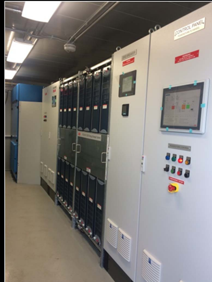
FESS module interior with PCS100 inverters
