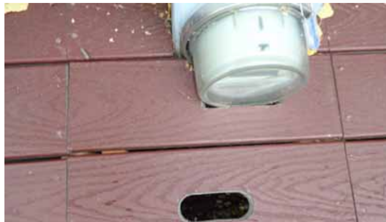
Sample Hazards / Obstructions
