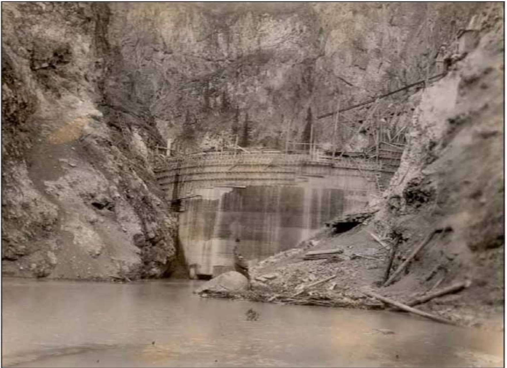
Figure 12. Upstream face of diversion dam under construction.
