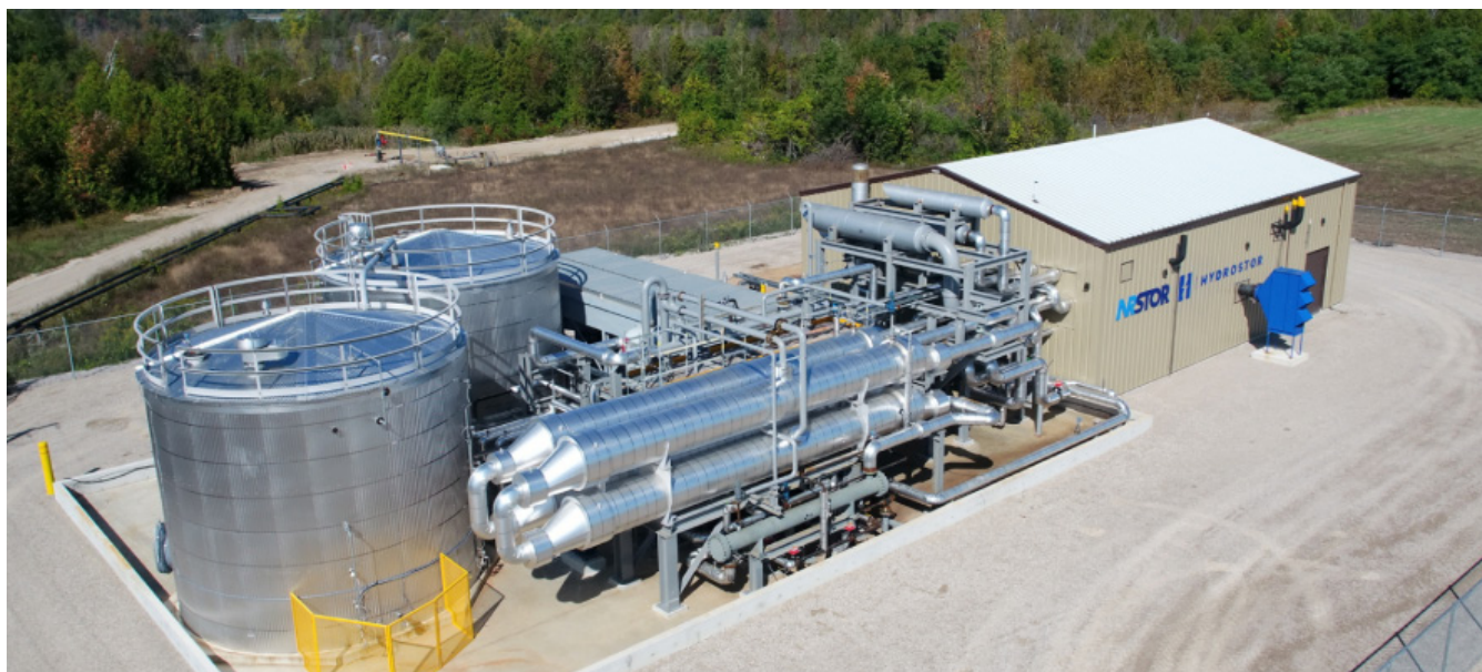
FIGURE 24 Hydrostor 2.2MW / 200MWh A-CAES facility in Goderich, Canada. 35
