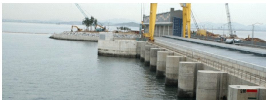
FIGURE 15 Sihwa Lake Tidal Power Station, located in Gyeonggi Province, South Korea, is the world's largest tidal power installation, with a total power output capacity of 254 MW.
