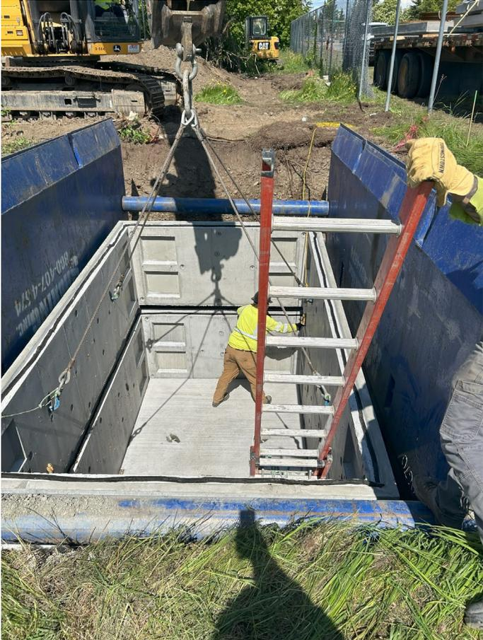
This project will relocate approximately 1.4 miles of existing overhead distribution and sub-transmission circuits underground, extending from the north side of East Northern Lights Boulevard to the north side of Brighton Park. Construction activities started in late May. Duct system has been installed, and conductor installation will start in November.
