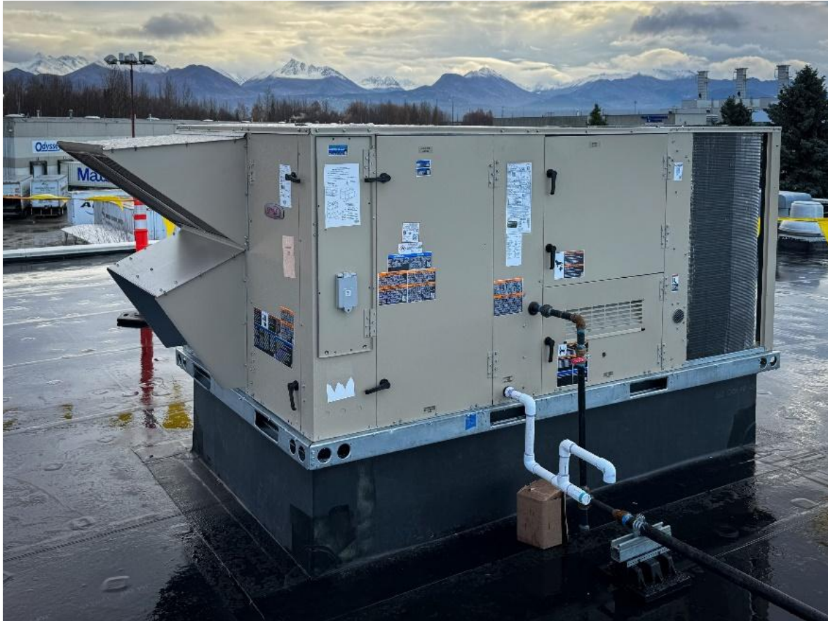
Figure 8: The air-source heat pump on the Annex building includes a gas furnace for backup/auxiliary heating.
