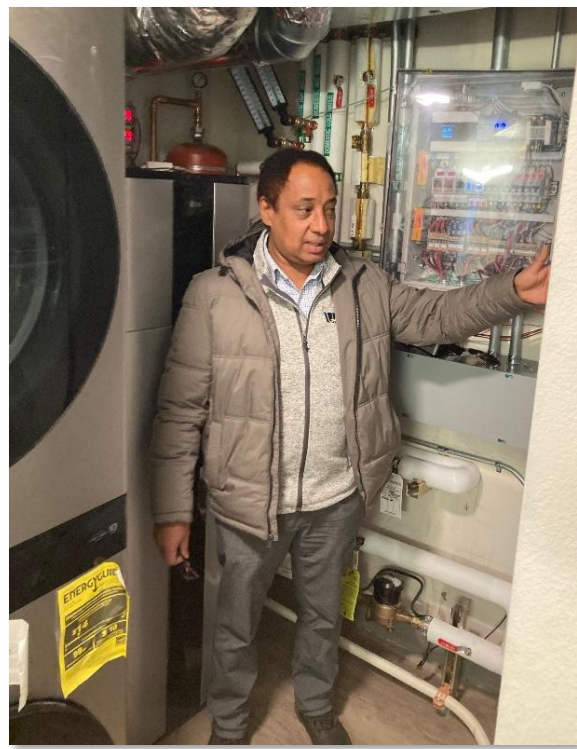
Figures 12 & 13: Dr. Getu Hailu showing the building energy monitoring system controlling the heat pump systems.
