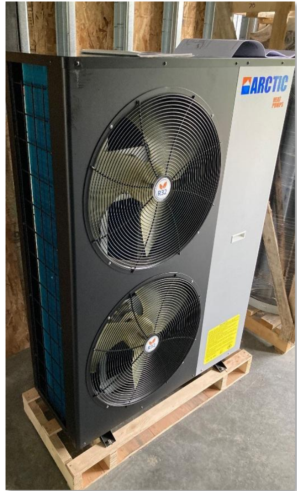
Figure 7: An air-to-water heat pump system preparing for installation. This system is rated to -31F.
