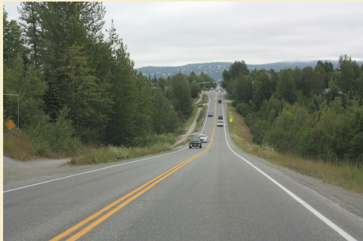
Chugach will be doing a series of distribution, subtransmission and transmission line activities along O'Malley Road between now and the end of the year.
