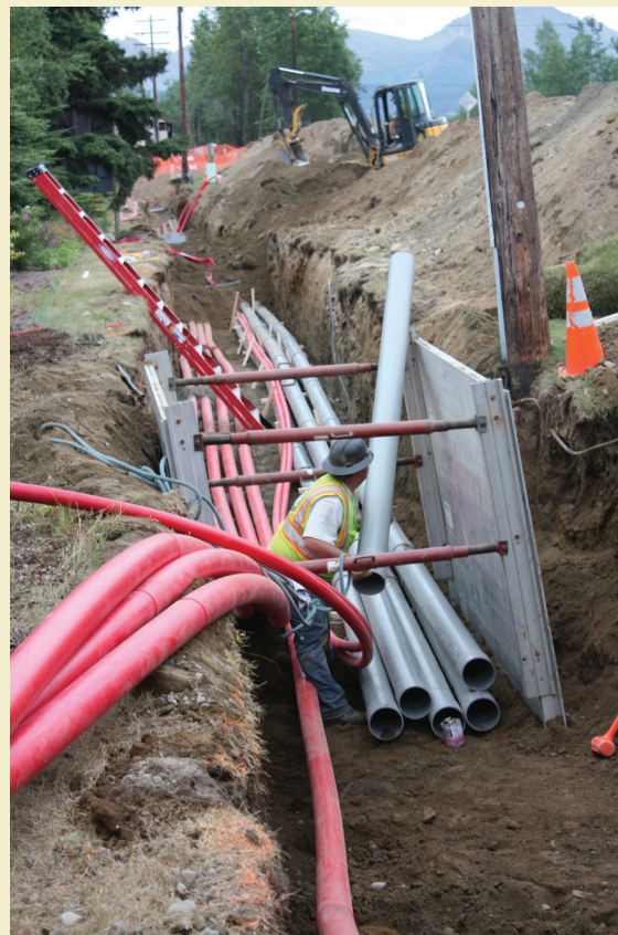
Conduits are being installed for both the new subtransmission and distribution circuits along O'Malley Road.
