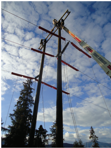
Several transmission line projects are funded in the capital budget.
