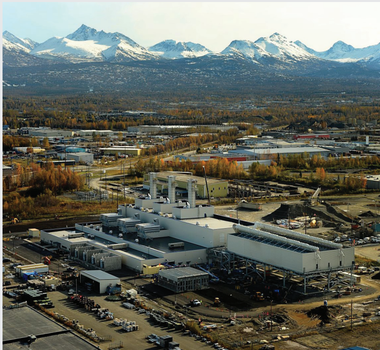
Construction and commissioning of the Southcentral Power Project is nearly complete. Commercial operation is expected in the first quarter of 2013.
