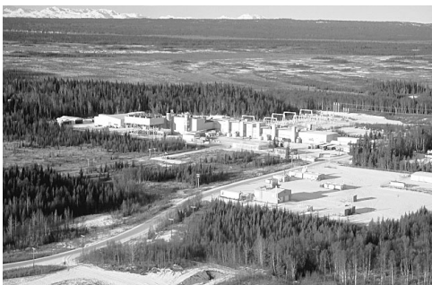
Beluga Power Plant
