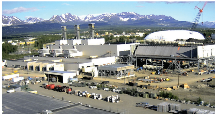
The gas turbines first firing at SPP will take place in August.
