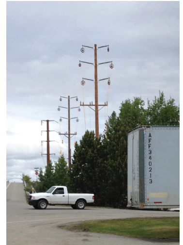
A short segment of new transmission line will connect SPP to the ML&P system.
