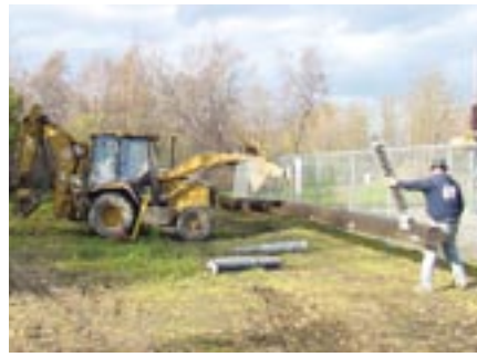
A Chugach contractor moves structure hardware out of the way at the new Postmark Substation.
