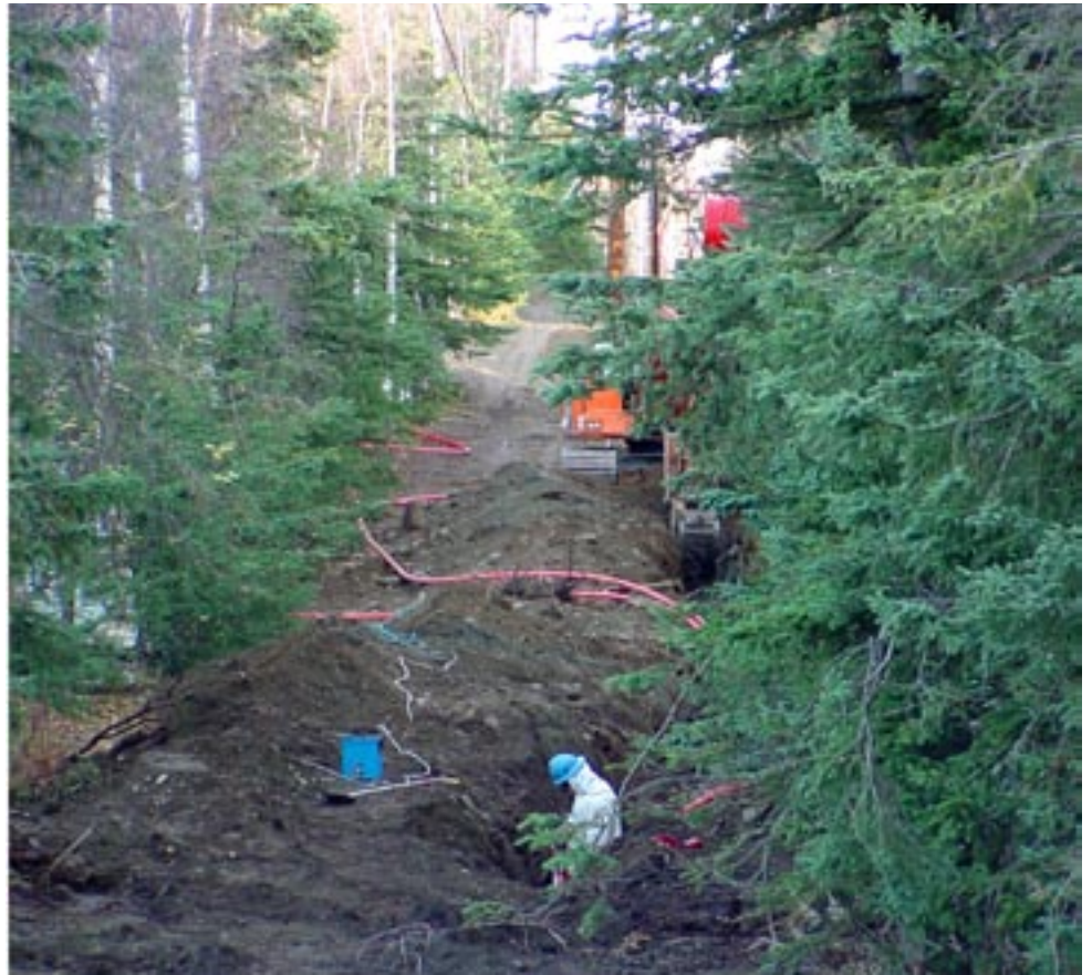
Chugach's contractor digs the trench for an overhead to underground power line conversion project near Rabbit Creek Elementary School.
