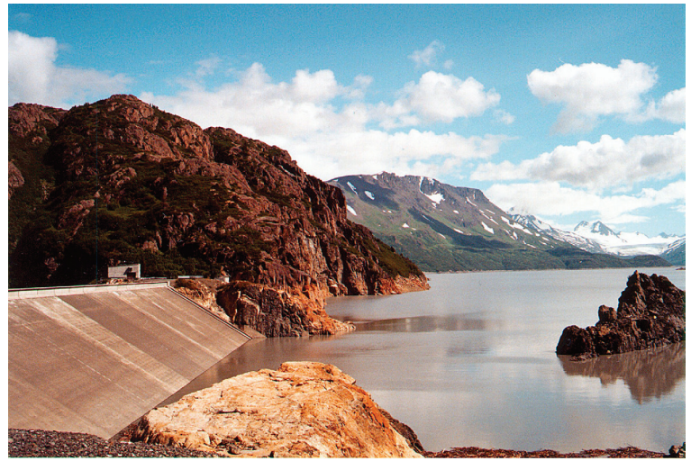
The reservoir at the Bradley Lake hydro project rose 13 feet in 7 weeks this fall.
