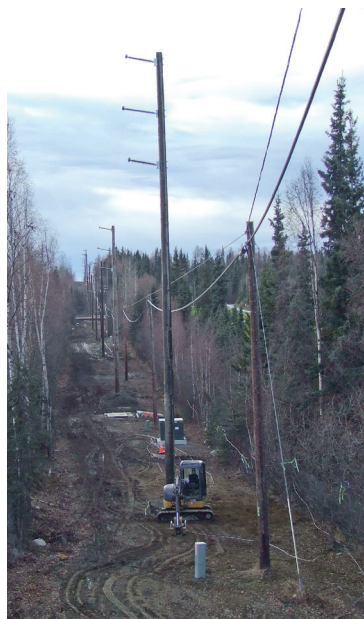
Poles have been set along O'Malley Road for the new 138-kv transmission line. To minimize the impact on private property (a neighborhood goal expressed during the years-long public process prior to construction) poles are located in the road right-of-way with all three conductors on the road side of the pole, thereby reducing the need for additional easement on adjoining properties. In this photo, taken alongside the Anchorage Golf Course near Elmore Road, the 12.5-kv electric lines and cross arms have already been removed from the former overhead distribution poles on the right. The shortened poles now hold only the telecommunications lines. Conduit for new underground telecommunications circuits were installed in the same trench where the new underground electric lines were buried.
