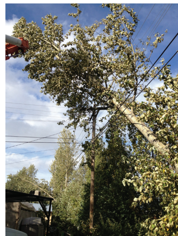
Trees falling into cleared easements caused most of the outages in September storms.
