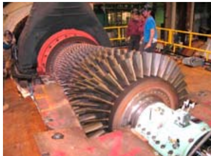
The crews pulled the Unit No. 6 turbine rotor for inspection during the overhaul. They inspected and cleaned the unit's blades.
