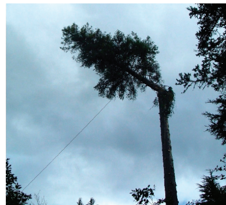
Chugach’s contractor uses a rope to guide the treetop safely to the ground.
