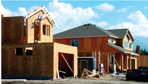
New houses are being built off Lake Otis between Huffman and O'Malley roads.
