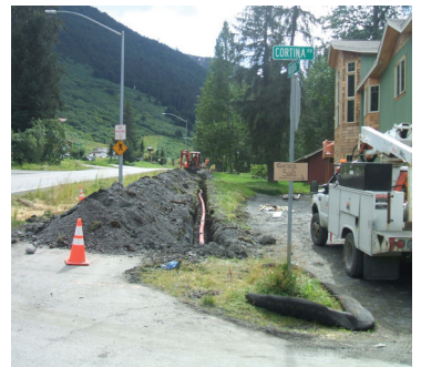
A new feeder tie along Arlberg Road is among several Girdwood projects Chugach is doing in 2012.
