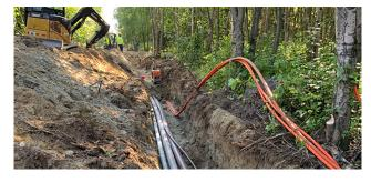
21 undergrounding fees. The effort included retiring approximately one mile of three-phase primary on the west side of Muldoon from Creekside to Northern Lights, and the trenching, boring, duct, vault, and conductor installation for a new underground distribution system. The project was finished in 2020 and landscaping will be completed in 2021.
