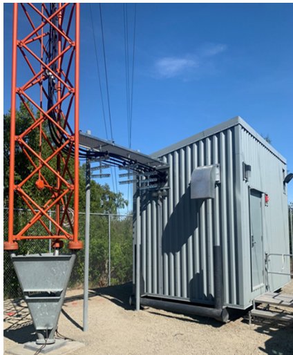
New Bernice Lake repeater shelter
