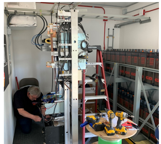
Interior equipment installation
