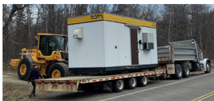
Original repeater shelter removed
