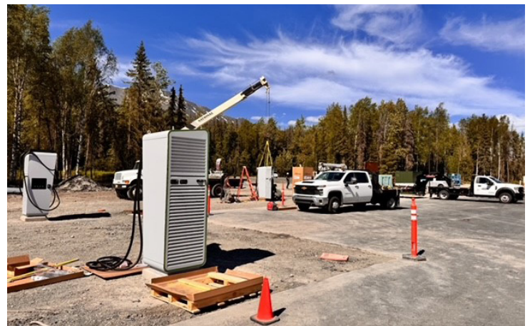
EV fast chargers being installed in Cooper Landing
