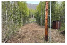
the importance of keeping the easements clear as fire breaks and possible evacuation routes. Chugach has other tools to use as well when the fire danger is high, including disabling automatic reclosing and, in extreme situations, preemptively shutting off power. {26835}
