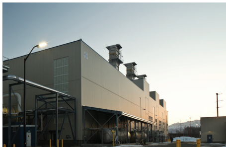
The CO2 emissions rate from the new Southcentral Power Project is much lower than from older natural gas-fired plants.
