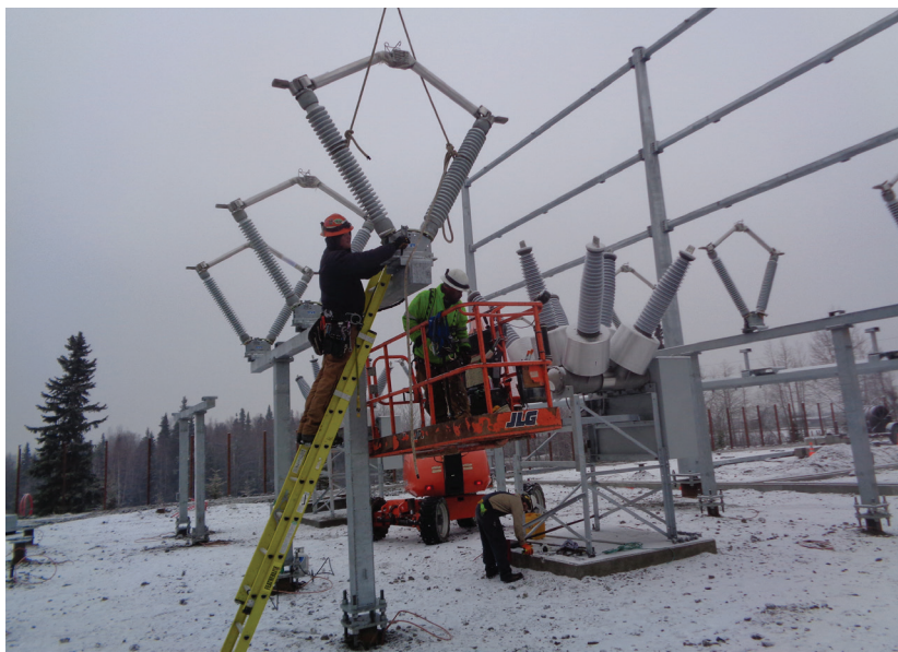
Construction continues on the Hane Substation along O'Malley Road.
