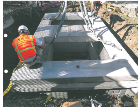
A new concrete vault near the Campbell Lake Substation was installed as part of a project to move power lines along Victor Road underground.
