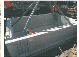
A new concrete vault near the Campbell Lake Substation was installed as part of a project to move power lines along Victor Road underground.
