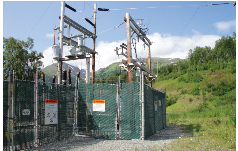
In July Chugach will begin a rebuild of the Hope Substation. The regional transmission system, as well as customers served by the substation, will benefit from the addition of remote switching capability.
