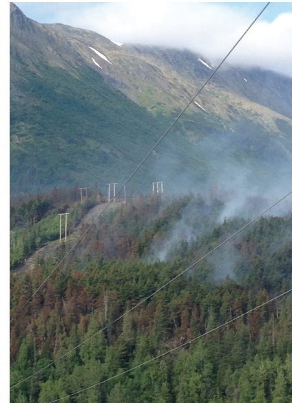
A wildfire in June temporarily halted work on the Stetson Creek diversion project at Chugach's Cooper Lake Hydroelectric Project. A section of 115-kilovolt transmission line between Sterling and Cooper Landing was de-energized for several days as firefighting efforts were underway.
