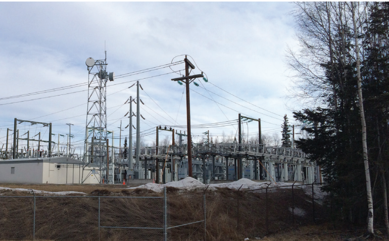
Communications infrastructure in some Chugach substations will be upgraded.
