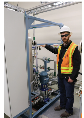
Project Engineer Andrew Laughlin explains the new and more efficient cooling skid at Daves Creek SVC
