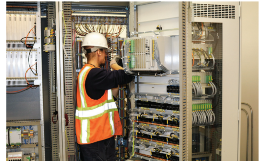
A worker terminates cable in the new control cubicle at the Soldotna SVC
