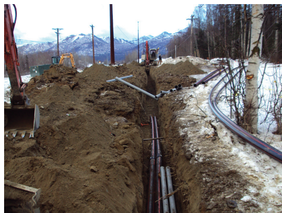
A Chugach contractor has been working through the winter on a project to convert overhead electric distribution lines to underground along the south side of Tudor Road between Elmore Road and Patterson Street.
