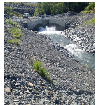
Stetson Creek diversion
