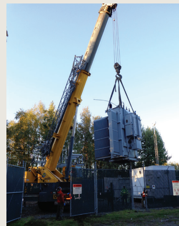
In mid-September crews moved a transformer out of the Turnagain Substation on Wisconsin Street. The old transformer is being replaced to ensure the continued reliability of the distribution substation that serves more than 4,200 metered-locations in West Anchorage. The transformer swap and related work will be completed by the end of the year.
