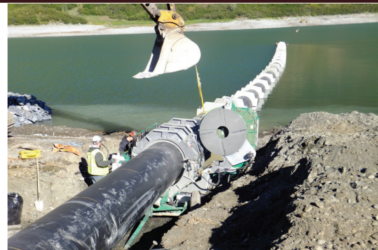
The discharge end of the diversion pipeline was floated onto Cooper Lake before being sunk into place on the bottom of the reservoir.
