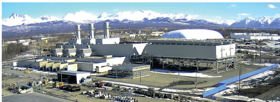
Southcentral Power Project
