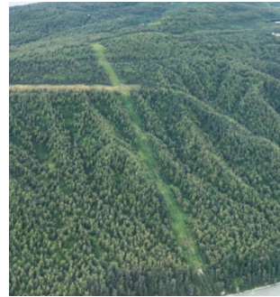
Transmission lines from the Susitna-Watana Hydroelectric Project will connect to the Alaska Intertie, a transmission line owned by AEA that runs between Willow and Healy.
