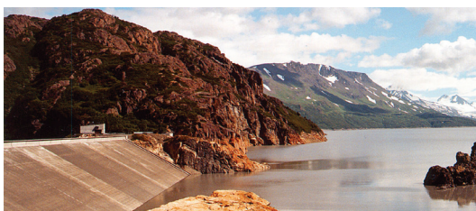
The Bradley Lake Hydroelectric Project reservoir supplies the water for a powerhouse on the shore of Kachemak Bay.
