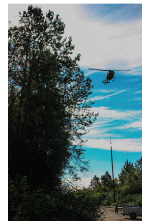
A helicopter was used to set the poles for a new distribution line crossing at the Chuitna River.
