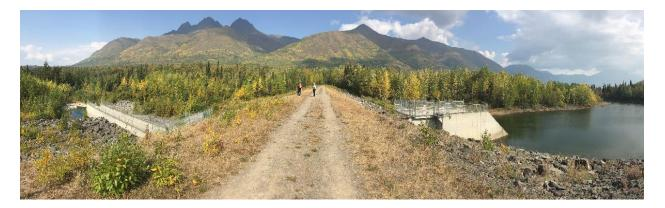
Figure 1-2. Dam crest and ungated overflow spillway, looking north.
